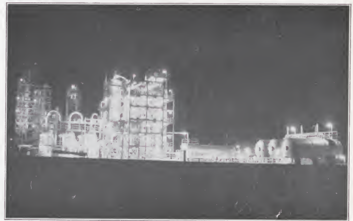
Stabilizing and splitting plant
